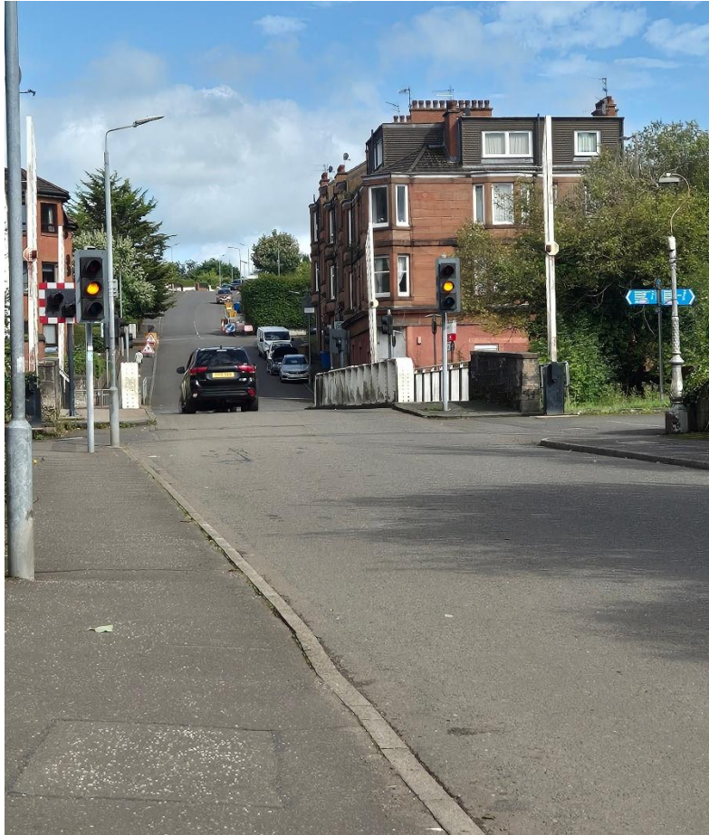
Pavement towards canal path – no dropped kerb
